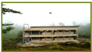
Yoshiko Hackett Primary Block (6-Unit classroom) construction
